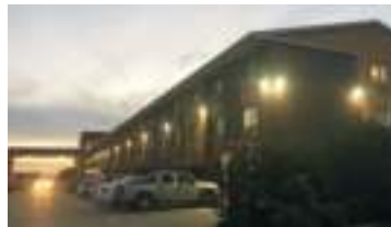
Parking lot lighting
